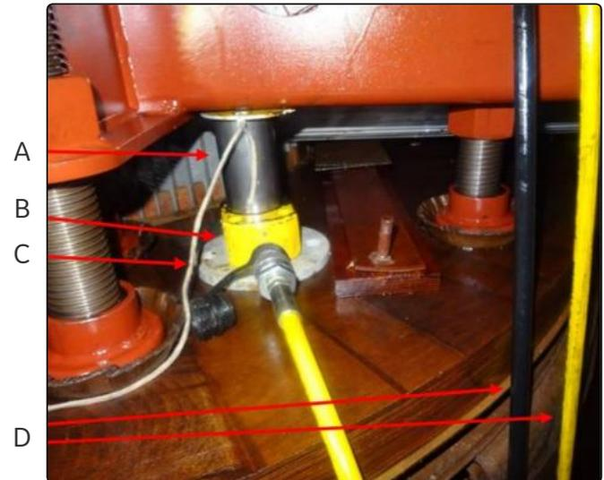
**Figure 5:** Example with one of the four hydraulic jacks in position between the clamping beam and the top winding platform, with load spreader to distribute the pressure. All four hydraulic lines were brought in through the HV turret.
