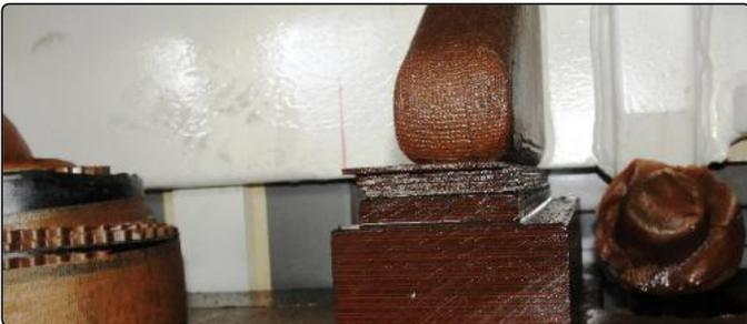
**Findings:** The clamping on one phase was found to be loose. The group of shims and thin block was so loose that it could be pulled out by hand.
