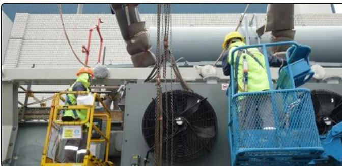
**Figure 4:** Improving cooling efficiency with upgrade of coolers and control cubicles on a 23 kV/435 kV three phases 420 MVA generator step up transformer.
