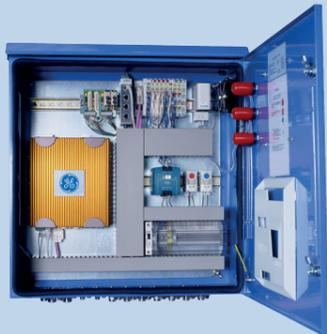
A modular and configurable system that can monitor the various key components of a power transformer listed here, depending on the asset owner's requirements.
