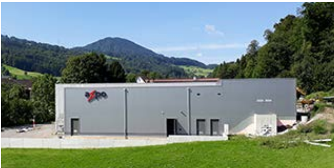
Figure 12: Axpo's Etzel substation in the Swiss Alps
