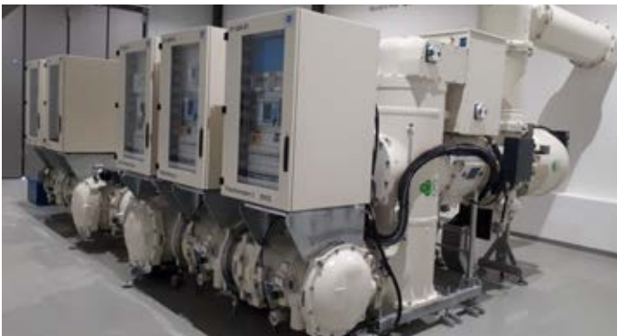
Figure 14: 123 kV GIS with g^3 installed and energized at Axpo's Etzel substation in 2018
