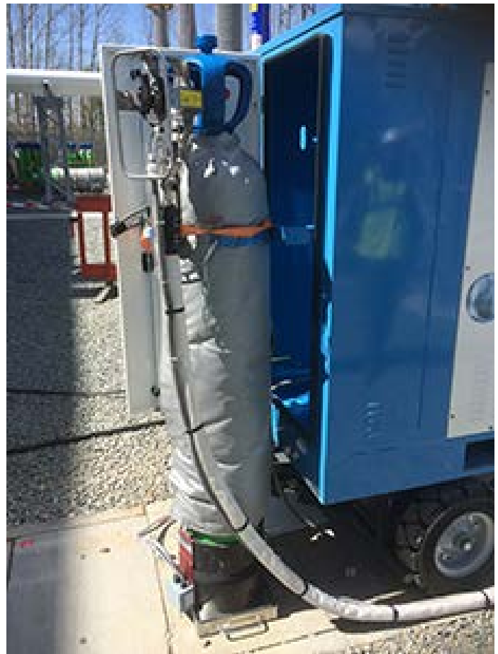
Figure 6: g 3 cylinder with warming system
