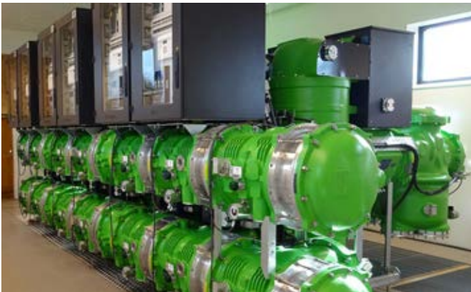
Figure 1: CERIOUS' F35-72.5 kV g^3 gas-insulated substation, including six circuit-breaker bays, is located in Denmark
