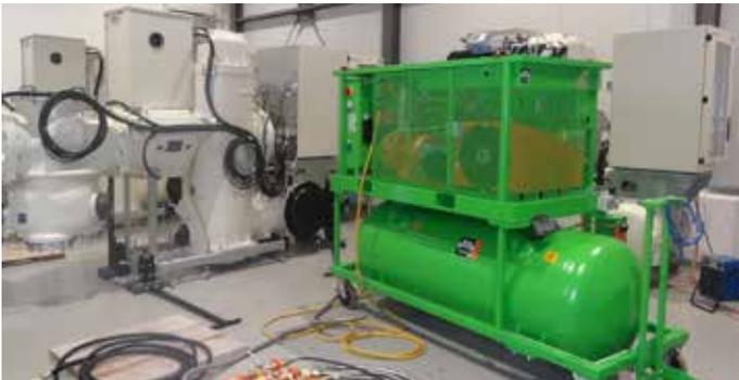
Figure 13: DILO's  $g^3$ -service cart used at Axpo's Etzel substation
