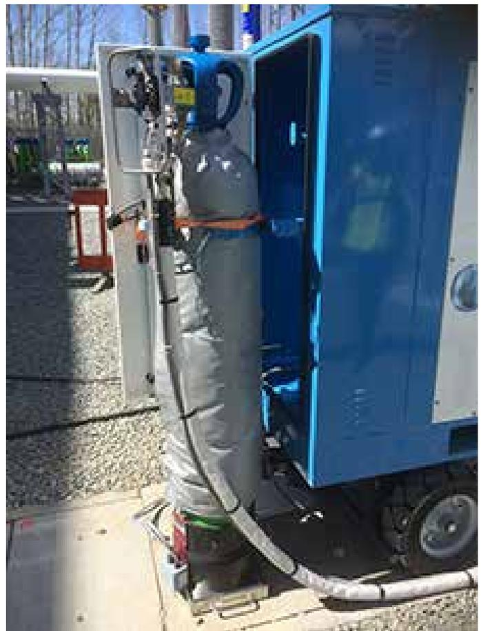
Figure 6: g<sup>3</sup> cylinder with warming system
