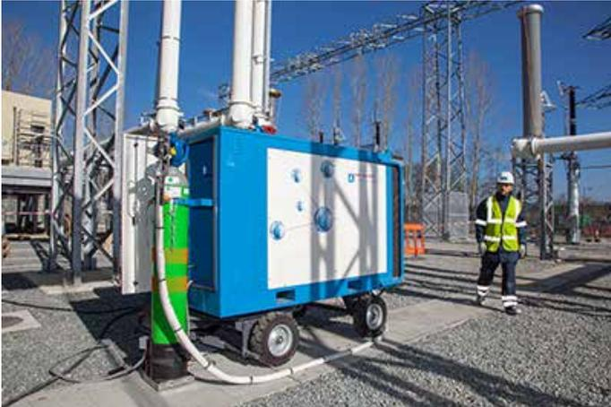
Figure 4: Air Liquide's g<sup>3</sup>-filling cart in service at a National Grid site in the UK
