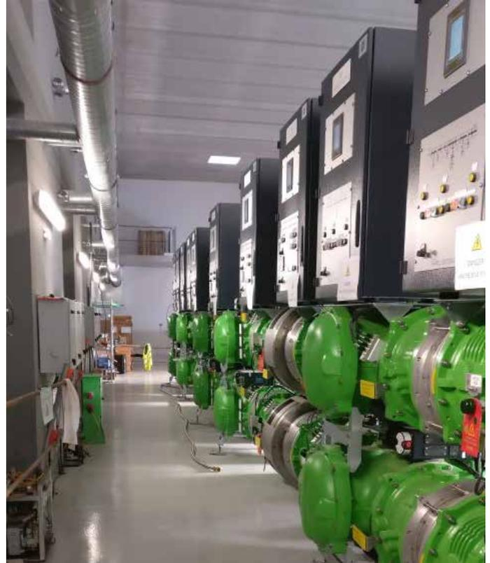
Figure 15: 72.5 kV F35 GIS using  $g^3$  installed in RTE's Grimaud substation in France
