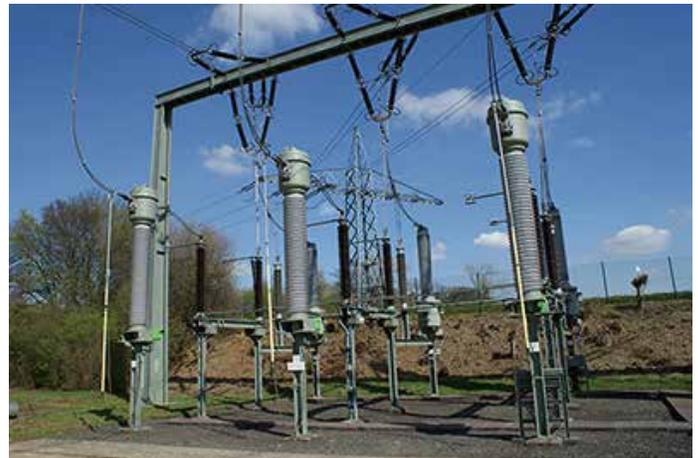
Figure 3: An  $SF_6$ -free 245 kV current transformer using  $g^3$  installed at a TenneT substation in Germany
