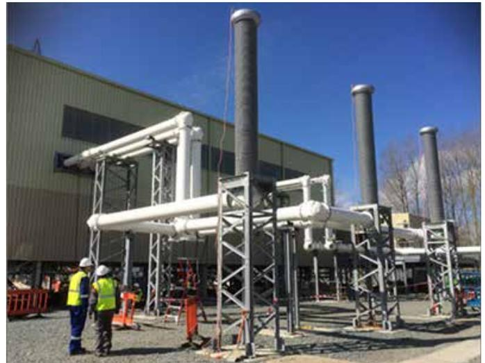
Figure 2: A 420 kV gas-insulated line filled with  $g^3$  at National Grid's new Sellinglee substation in the UK
