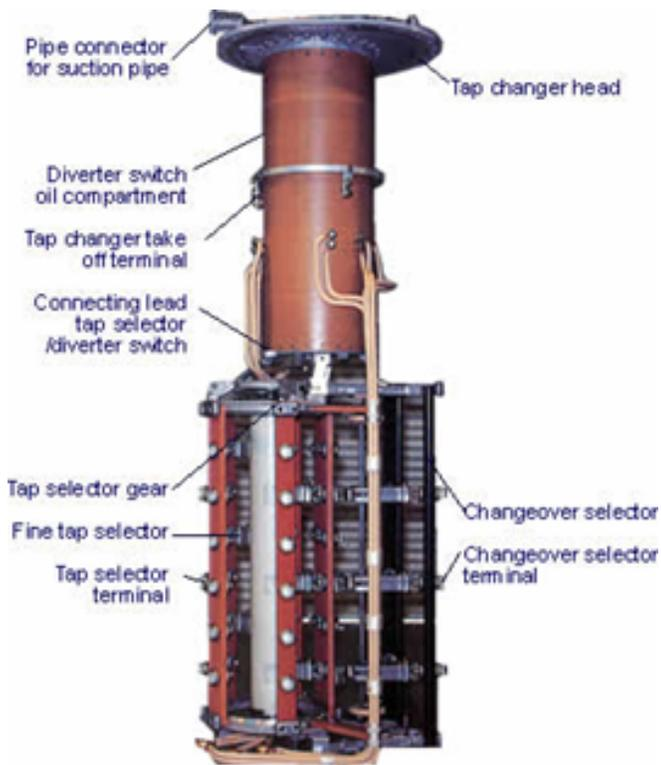
The transformer tap changer is a vital part of the transformer and needs to be monitored to ensure correct operation.
