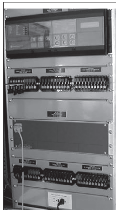
Fig 4. New Feeder Protection and Control Panel Layout.
