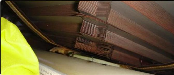
**Findings:** Short circuit and circulating current damages identified on core and core frame of a 19 year old large step down transformer 230 kV/10,5 kV.
